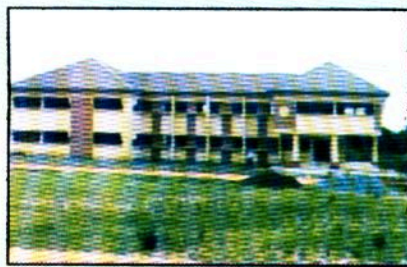
New Project Management Building
