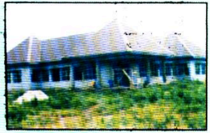
ICT centre donated by Zinox Technologies under construction
