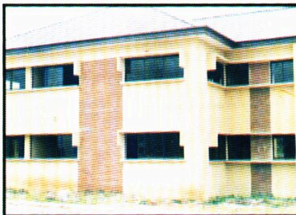
A view of the Project Management Building also commissioned by the VC, Prof. C.O.E. Onwuliri on 27th Sept. 2006.
